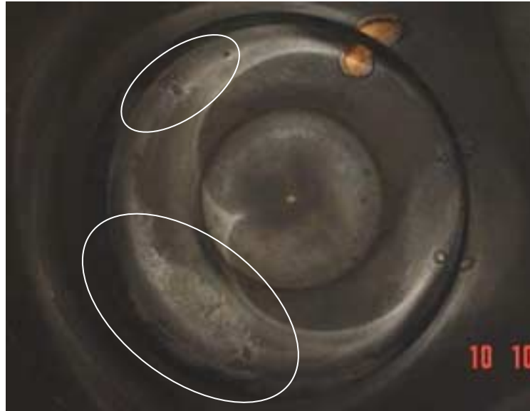
Picture 1 – Faulty Injectors on Unit 10 corresponding to high Vanadium and Iron in Fig 5.
